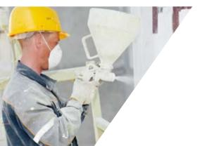
Silfoam offers an innovative and easy way for applying aerogel insulation. This product can be easily sprayed or applied with plaster tools on small or large complex structures.
